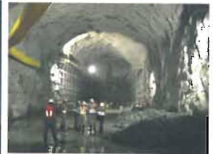
Montañas hydroelectric generation project. Don Matías, Antioquia.
